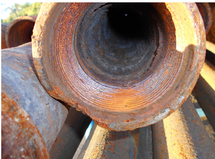
Figure 2. Further analysis of the area with 100% wall penetration.
